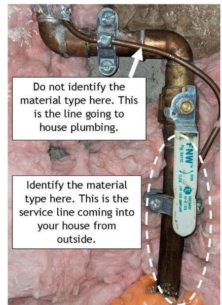
2. **Do a scratch test:** Gently scrape the pipe using a coin or the flat edge of a screwdriver to reveal the metal. Do not use a knife or sharp object. If the pipe is painted, gently sand or scrape the paint away first to expose the metal.
